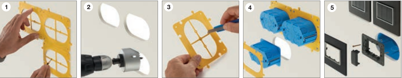
1. and 2. Use the V71573 accessory as a template for a precise drilling. 3. Remove with a cutter or scissors the central grid. The accessory can also be used as a tie. 4. When box positioned, fix it to the hollow wall with screws for plasterboard. 5. The result is a flush profile.
