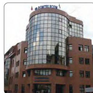
Name: ROMTELECOM OFFICE BUILDING Country: Romania
