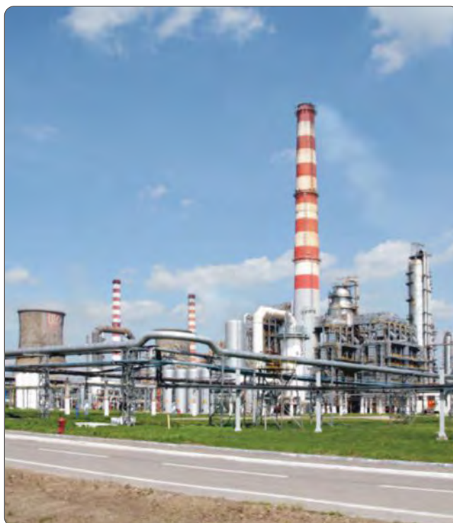
Name: LUKOIL RAFINERY PLOIEȘTI Country: Romania
