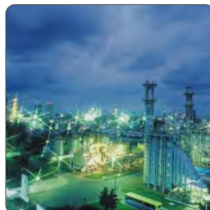
Name: PETROM BRAZI POWER PLANT - REHABILITATION Country: Romania
