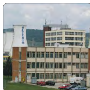
Name: OLTCHIM - REHABILITATION Country: Romania
