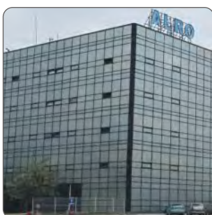
Name: ALRO - REHABILITATION Country: Romania
